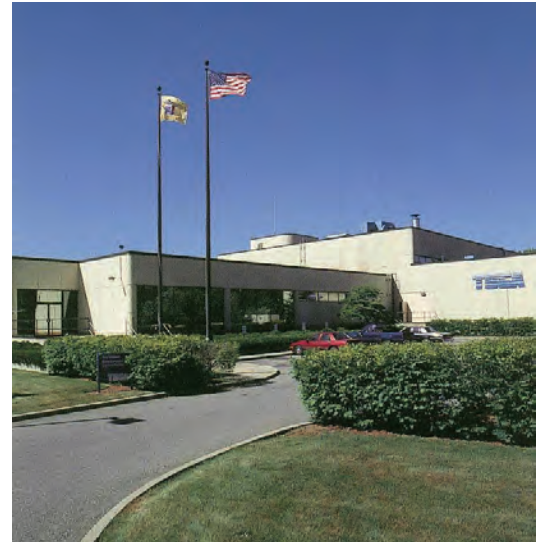
Today, TBSA operates at its original design capacity of 7.5 million gallons per day (MGD). The potential plant capacity is rated for 10 MGD.
